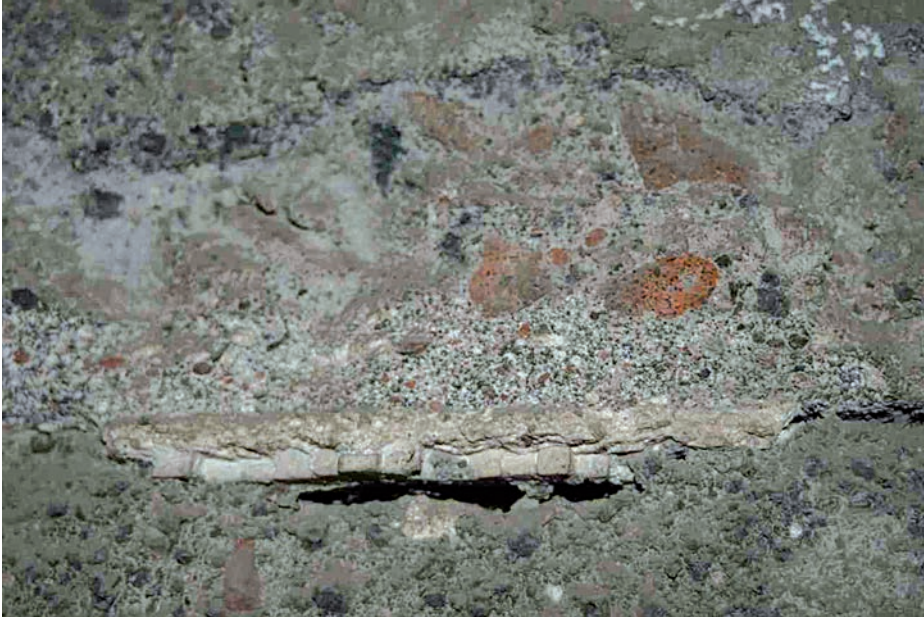
Fig. 3. Large fragment of a mosaic floor (upside down) embedded in a wall of a Pompeian building as recycled material. The stratigraphy of the preparatory layers of the mosaic, containing abundant ceramics fragments, is on display.
