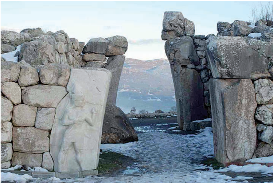
Fig. 1. Megalithic fortified walls of Hattusa, the ancient capital of the Hittite empire. They are composed of shaped limestone blocks with no use of binder.
