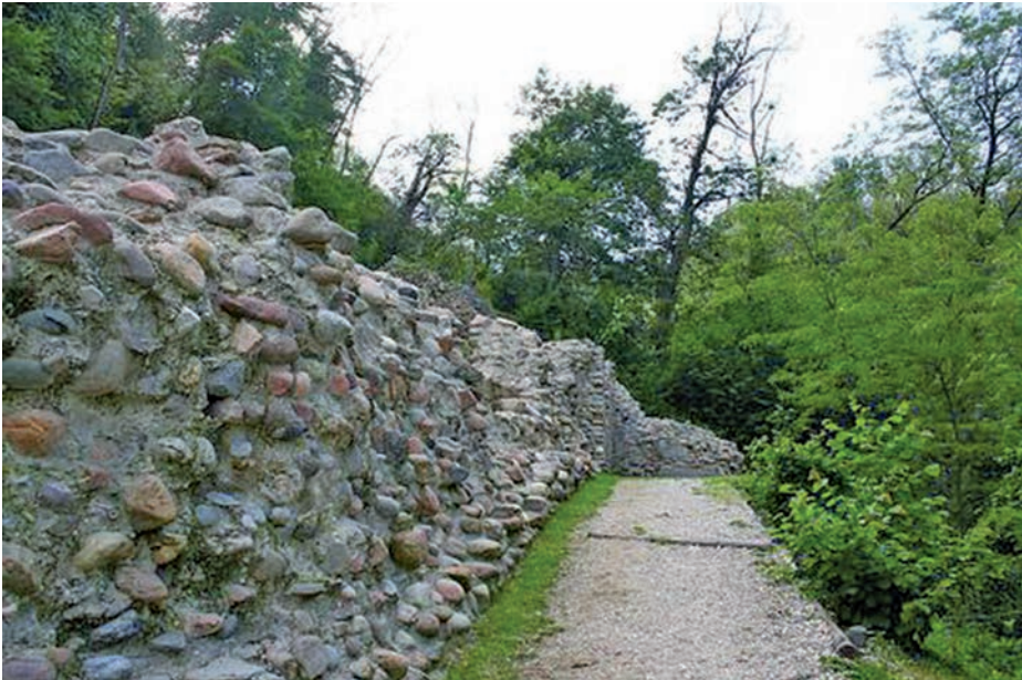
Fig. 2. Typical infilling of the large wall structure of a Roman fort by opus caementicium , containing fragments of rocks and broken ceramics embedded in the lime matrix.
