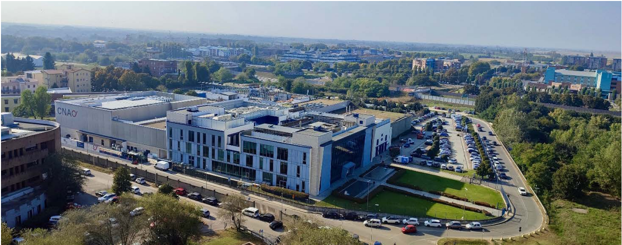
Fig. 5. Photo of CNAO from the nearby San Matteo hospital.
